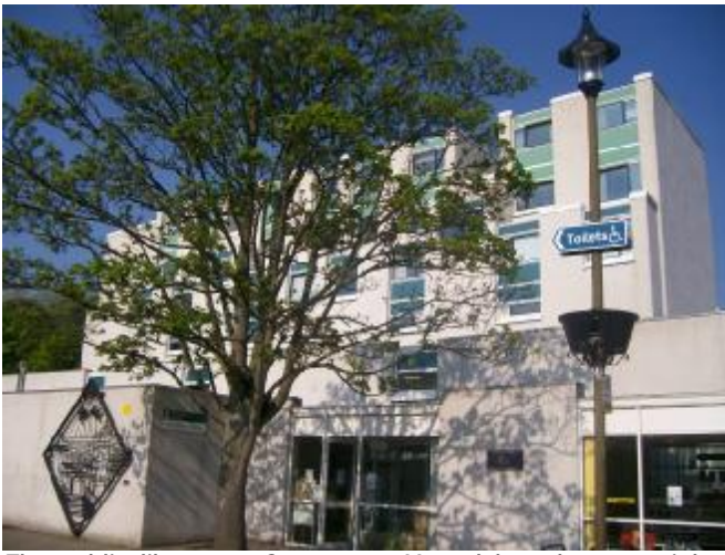
The public library at Guyancourt Vennel has the potential to provide a sound basis around which the regeneration of the area as a centre for specialist retailing could be pursued.
